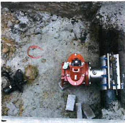
Water Main Installation
