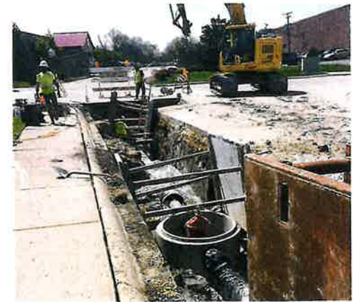
Water Valve Installation
