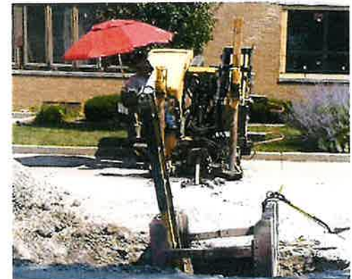
Water Service Installation
