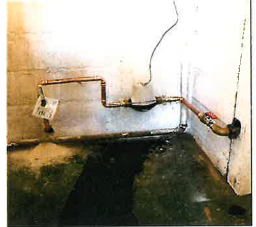
Water Meter Installation
