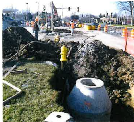
Fire Hydrant & Valve Installation
